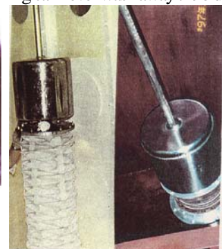
(a) New Condition (b) Used for 4 Years Fig.7 Floating High Suction System
